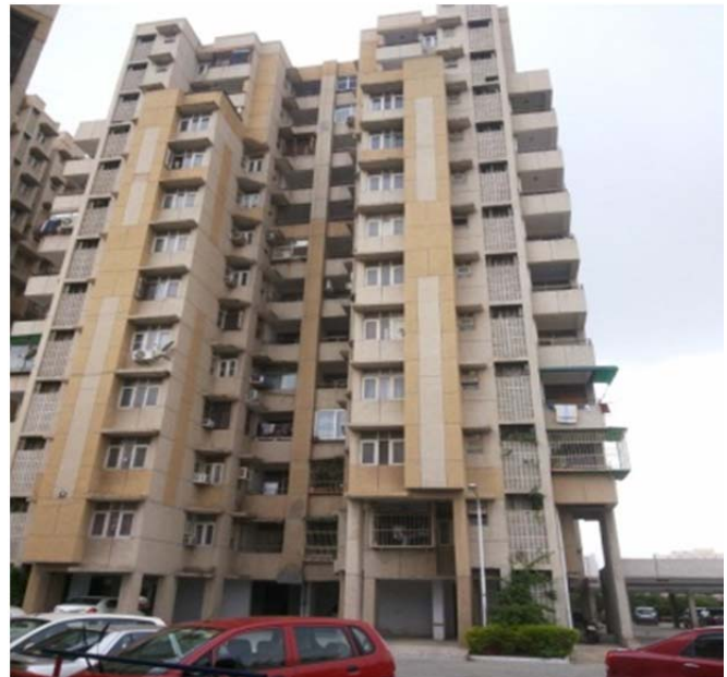
Slide 2: Image of typical high rise residential development in Gurgaon with stilt/podium parking. (source: Author)
